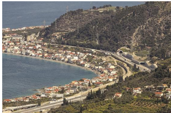
OLYMPIC FEAT The Olympia Odos roadway concessionaire ceased construction for two years as stakeholders hashed out new terms.
